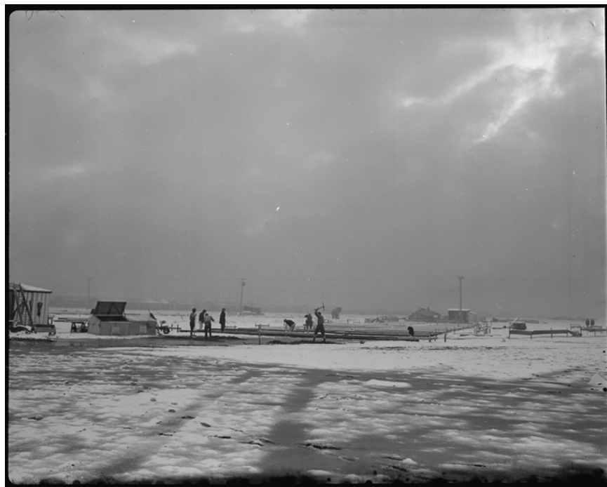
Tule Lake Relocation Center, Newell, California. A wintry view of early construction work on the Tule Lake schools. All work is done by the internees.
